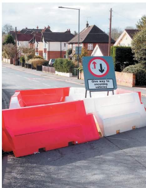
Speed bumps are to be installed on Courthouse Road, Maidenhead. Ref:133365-5
